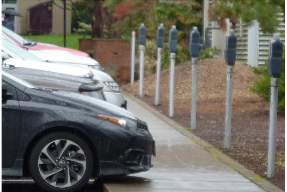
Figure 52: Circulation along the sides of Lot H is non-compliant in key areas. This central circulation path is impacted by adjacent parking and does not meet accessibility requirements.
