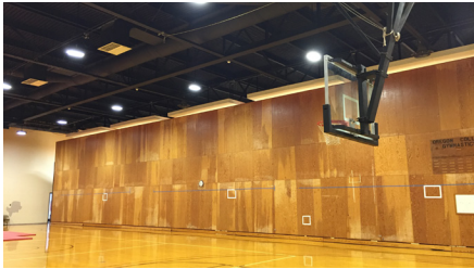
Figure 42: The two gymnasium spaces are separated by a bank of retractable seating. With no acoustic separation, they cannot effectively be used at the same time.
